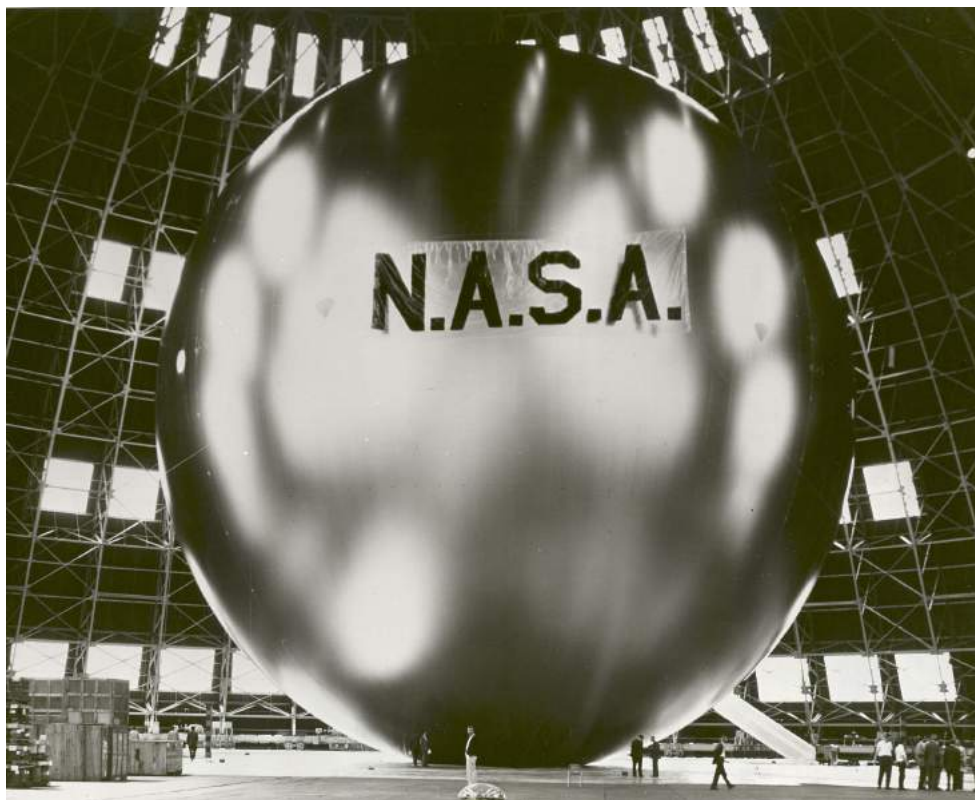
Echo 2 satellite, lifted to \sim 1,000 km orbit
